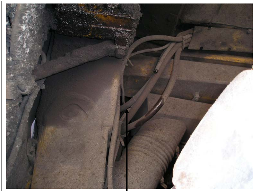
Hoses from cab running over to left side of engine.
